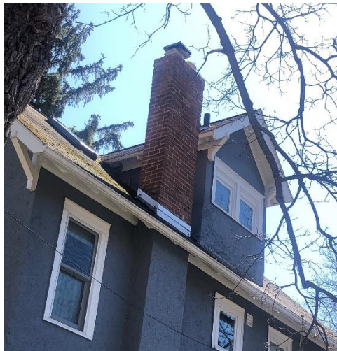
Fig. 43. Photograph by Claire Buchinger. Biological Growth, West Façade . April 2, 2023. Ithaca, New York.
