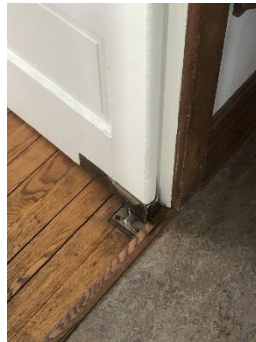
Fig. 24. Photograph by Claire Buchinger. Dining Room to Kitchen . February 25, 2023. Ithaca, New York. Fig. 25. Photograph by Claire Buchinger. Butler Door Pivot Hinge . February 25, 2023. Ithaca, New York.
