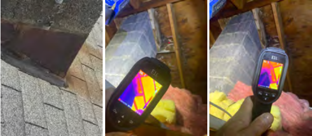
5. North Chimney Chimney Flashing: Tar covered - Previous leakage noted seal flashing recommended
