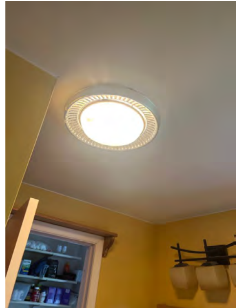
2nd Floor Bathroom
