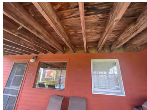
1st Floor Porch Roof
