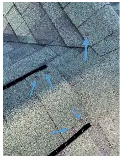
Middle of roof cap
