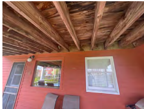
1st Floor Porch Roof
