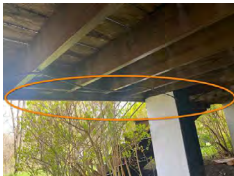
All south and east deck
