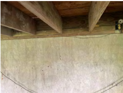
All Ledger Boards on the house
