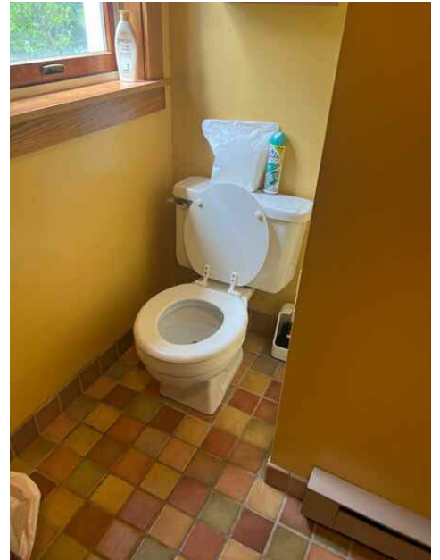
2nd Floor Bathroom
